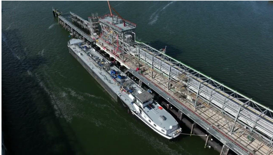
Jetty 7 Koole Terminals Botlek
