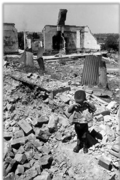
© Magnum Photos (Pinterest). Sophiatown House Demolition, Johannesburg, South Africa, 1961
